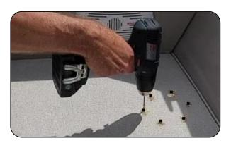
**14.** Lift the floor and check if there are conflict with the bolts. If some holes drilled in step 13 are in aluminum studs, enlarge those holes with a  $\frac{1}{2}$  " drill bit to make clearance for bolts and nuts.
